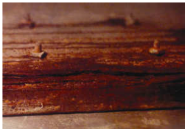
Fig. 3 - Brass tile clips.
